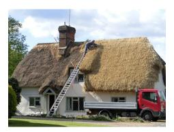
Most properties in the UK use either long straw, wheat reed or water reed. Many thatched properties are listed and when re -thatching is needed there is a requirement to use the same type of material as before.
